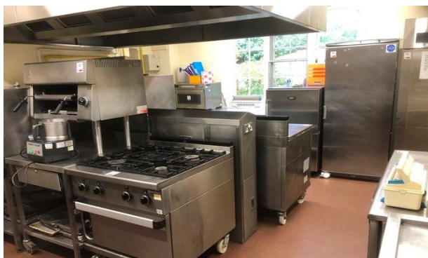
Commercial Kitchen Equipment
