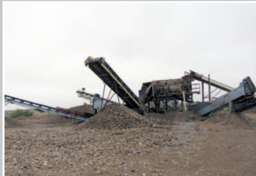
View of Wash Plant
