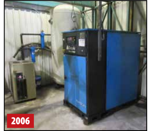
COMPAIR L55G-9A 75 HP AIR COMPRESSOR
