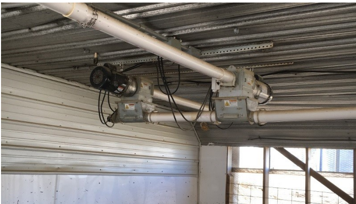
Incoming Feed Lines to Feeder Line
