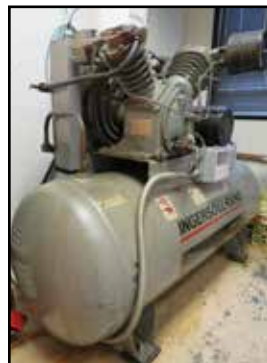
INGERSOLL RAND 10 HP AIR COMPRESSOR
