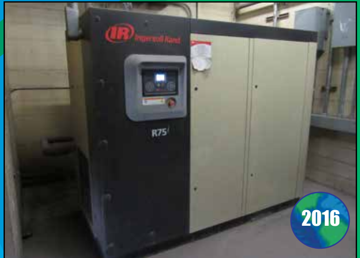
INGERSOLL RAND 100HP ROTARY SCREW AIR COMPRESSOR
