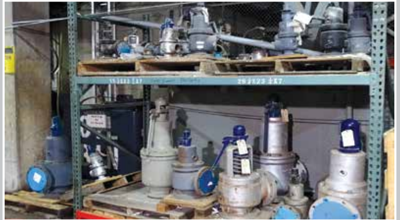
View of Valves
