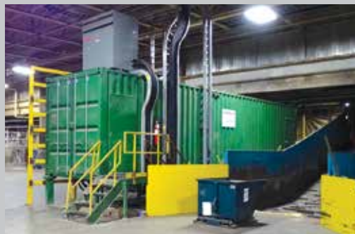
New Electronics System Enclosed Trailer
