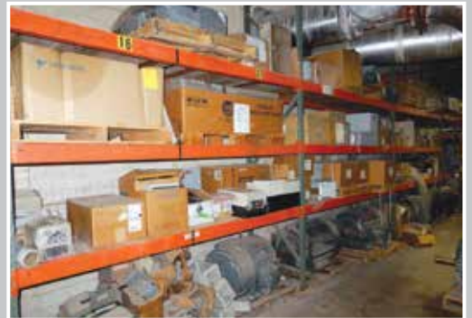
View of Electrical Spares
