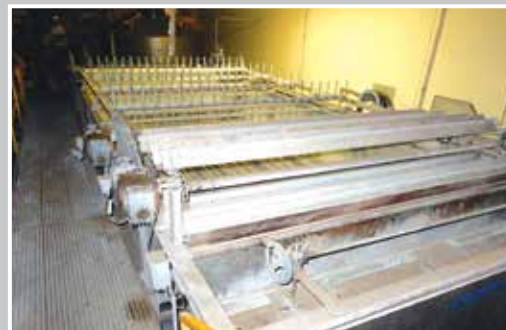
POSIDEN Dissolved Air Flotation Clarifier
