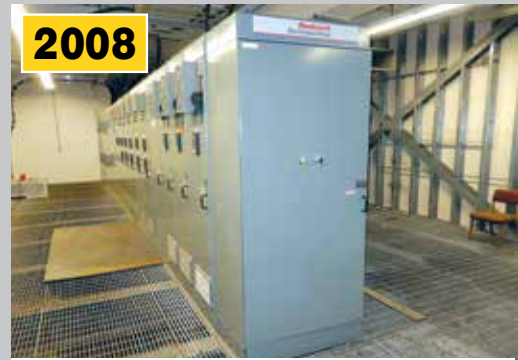
Rockwell Automotive Drives of PM3
