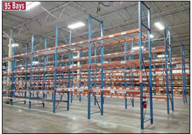
(95) Bays of INTERLAKE Tear Drop Pallet Racking
