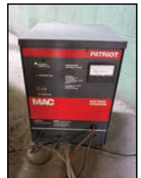
MAC Battery Charger
