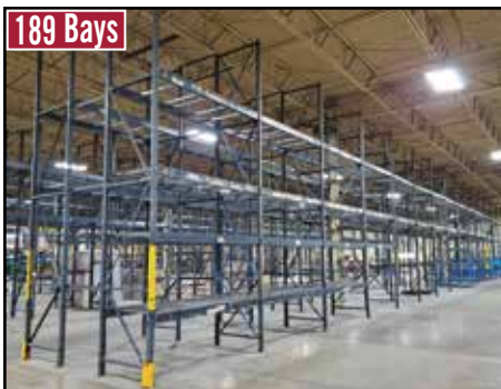
(189) Bays of RIDG-U-RAK Slot-Style Pallet Racking
