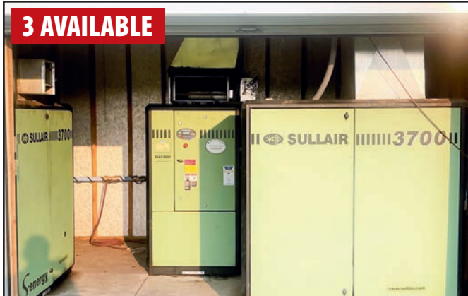
VIEW OF SULLAIR 55 HP AIR COMPRESSORS
