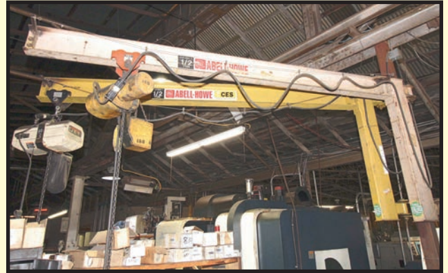
(APPROX. 6) ABELL-HOWE 1/2 T. CAP. WALL MOUNTED JIB CRANES
