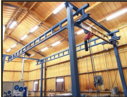
GORBEL 4,000-LB. CAP. GANTRY CRANE SYSTEM
