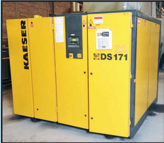
KAESER MDL. DS171 ROTARY SCREW AIR COMPRESSOR
