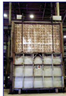
E4, 2100 Deg. F North American Mfg. Furnace, 170" W x 117" H x 140" D, natural gas, 6 burners, fiber lined, Honeywell controls
