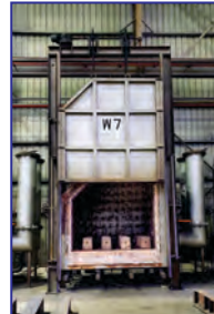
W7, 1850 Deg. F, 97" W x 58" H x 86" D, natural gas, 2 burners, fiber lined, Honeywell controls
