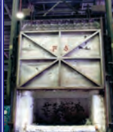
F3, 2200 Deg. F, 160" W x 118" H x 106" D, natural gas, 4 burners, fiber lined, Honeywell controls
