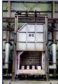
W6, 1850 Deg. F, 97" W x 58" H x 86" D, natural gas, 2 burners, fiber lined, Honeywell controls
