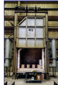
W9, 1850 Deg. F, 98" W x 68" H x 82" D, natural gas, 2 burners, fiber lined, Honeywell controls
