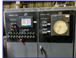
(above) East Side, 2500 Deg. F Custom Built Car Bottom Furnace, 216" W x 180" H x 300" D, natural gas fired, 10 burners, 2 zones, fiber lined, Honeywell controls with PLC
