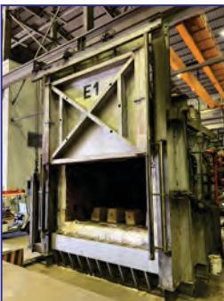
E1, 2100 Deg. F, 98" W x 62" H x 108" D, natural gas, 4 burners, fiber/brick lined, Honeywell controls
