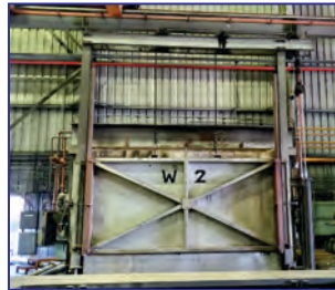
W2, 1850 Deg. F, 166" W x 76" H x 94" D, natural gas, 4 burners, fiber lined, Honeywell controls
