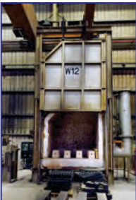
W12, 1850 Deg. F, 98" W x 68" H x 82" D, natural gas, 2 burners, fiber lined, Honeywell controls
