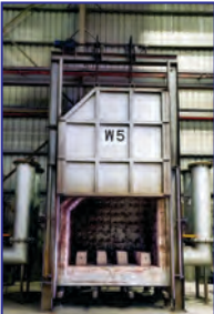
W5, 1850 Deg. F, 97" W x 58" H x 86" D, natural gas, 2 burners, fiber lined, Honeywell controls
