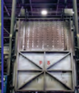
F5, 2200 Deg. F, 160" W x 118" H x 106" D, natural gas, 4 burners, fiber lined, Honeywell controls
