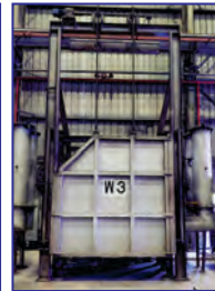
W3, 1850 Deg. F, 96" W x 61" H x 86" D, natural gas, 2 burners, fiber lined, Honeywell controls
