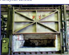
F1, 2200 Deg. F, 160" W x 80" H x 106" D, natural gas, 4 burners, fiber lined, Honeywell controls
