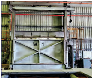
W1, 1850 Deg. F, 166" W x 76" H x 94" D, natural gas, 4 burners, fiber lined, Honeywell controls
