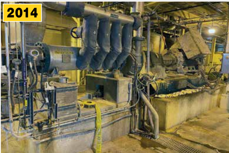
CELLWOOD Hot Disperser System
