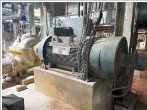
Pumps and Valves
