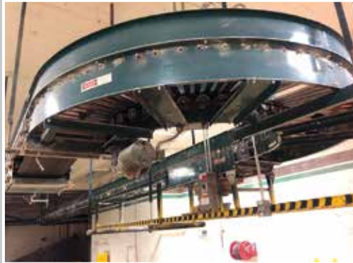
Large Quantity of Various Conveyor
