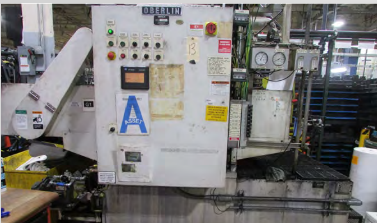
OBERLIN OPF-07 32" PRESSURE FILTRATION SYSTEM
