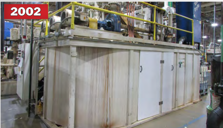
2002 OBERLIN PRESSURE FILTER OPF-18 PRESSURE FILTRATION SYSTEM
