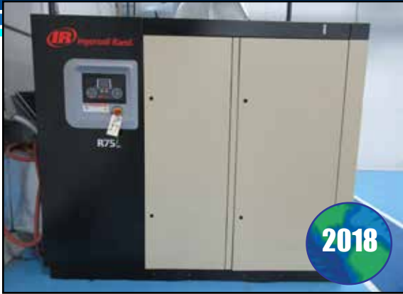
INGERSOLL RAND R75I-A125 100 HP ROTARY SCREW AIR COMPRESSOR
