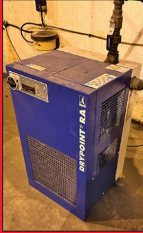
(2) BEKO Air Dryers (New as 2015)
