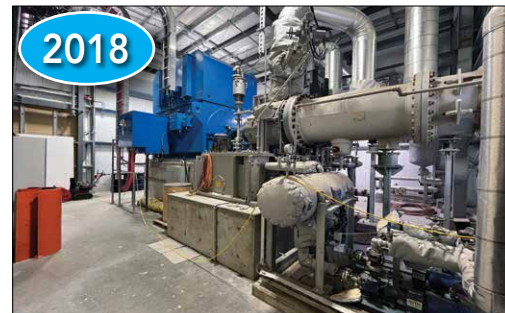
Howden Turbine Generator Twin Series Dual Casing Turbine SST-110 6.9 MW Capacity
