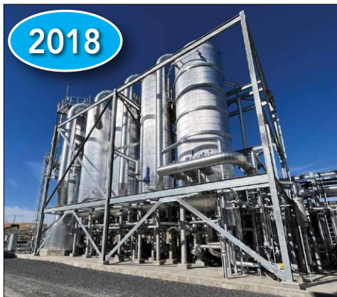
Rosenblad Design Group, Inc. Multi-Effect Evaporator System, Manufactured 2018
