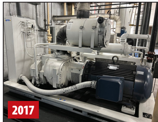
GARDNER DENVER ELECTRA-SAVER 200 EAU99U 200 HP COMPRESSOR
