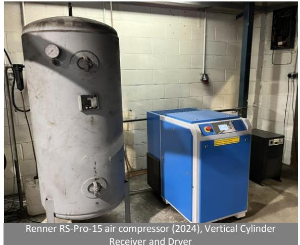
Renner RS-Pro-15 air compressor (2024), Vertical Cylinder Receiver and Dryer
