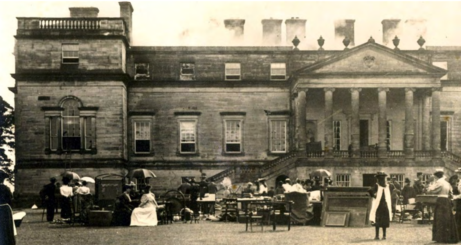
Above: Photographs from family records showing the efforts to remove the contents of the house to the lawn before they could be consumed by the fire.
