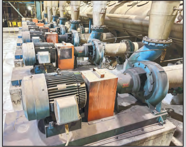
(6) GOULD 316 SS CENTRIFUGAL PUMPS WITH MULTI-DISC FILTER
