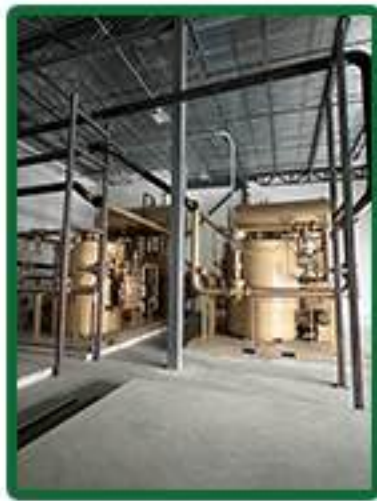
(2) 2022 Fulton FT-1000CU-LE Boilers, Hot Oil, Fuel Input BTU/HR 11,494, Heating Element Gas Fired, Heating Surface 907.2 sq/ft
